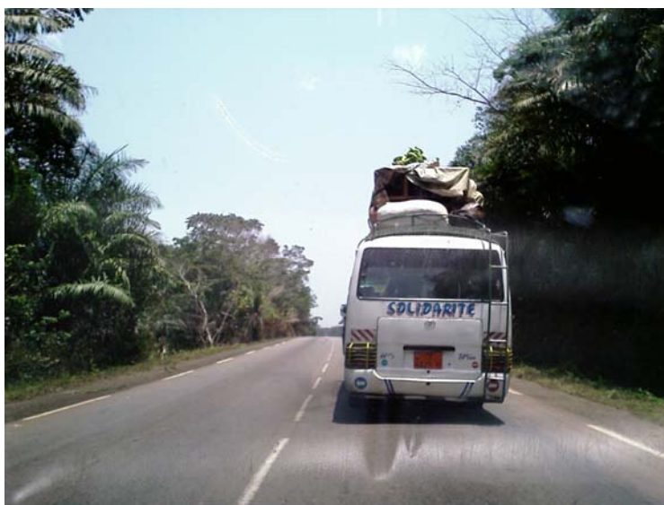
Figure 19: The Douala-Yaounde highway with fibre buried on the left hand side
